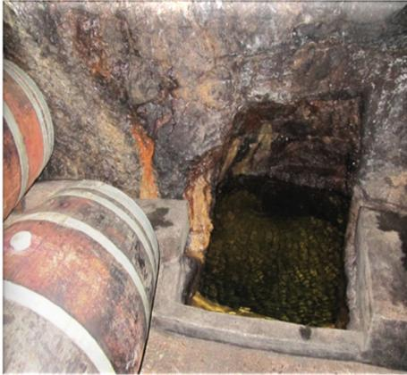
Natural climate control is used for those wineries that do not require any installation for the control of temperature and humidity, particularly in the aging areas, both in the barrel and the bottle rooms.
